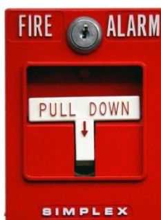
Figure 5 Fire Alarm Pull Stations of Mahamakut Building
