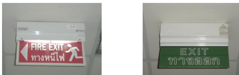
Figure 7 Fire Exit and Evacuation Route Signs of Mahamakut Building
