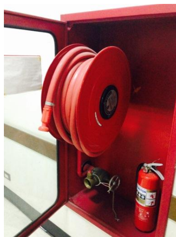
Figure 2 Fire hose reel at Mahamakut Building
