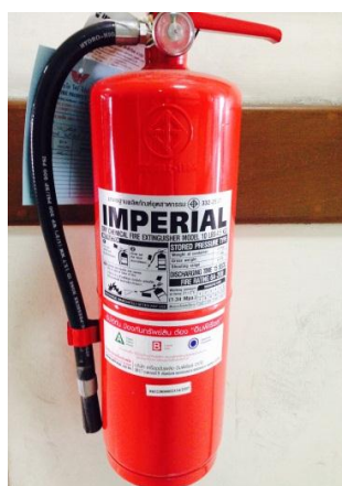
Figure 1 ABC Dry Chemical Powder Extinguisher used at the Department of Chemistry
